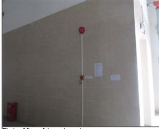
Photo of fire safety equipment Fire alarm.JPG
